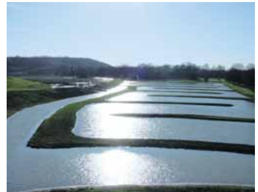
The lagooning in Harnes completes the wastewater purification process and provides high-quality water for a swimming pond. The photo shows the sedimentation pools.
