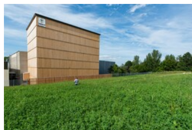
© Trench Austria GmbH
