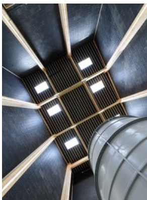
© Trench Austria GmbH
