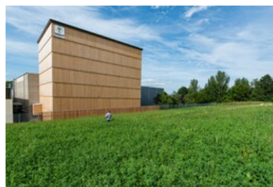
© Trench Austria GmbH
