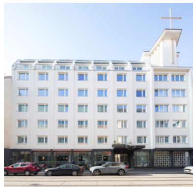
© BWM Designers & Architects
